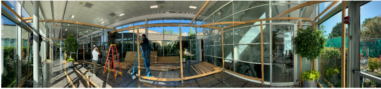
The Indoor Sukkah Under Construction
